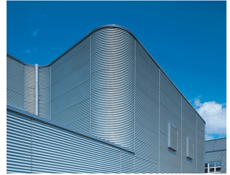
Multisport Complex, Walferdange, Luxembourg
